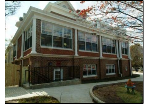
Main Building, Side View of Addition
