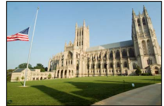
One of the largest Intensive Green Roofs in the metropolitan area
