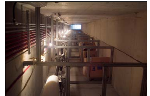
Interior of Utility Corridor
