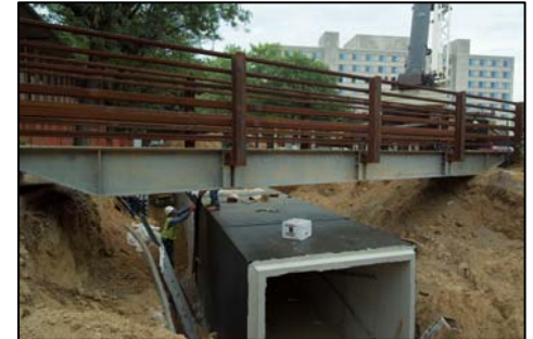
Temporary Pedestrian crossing over the Utility Tunnel
